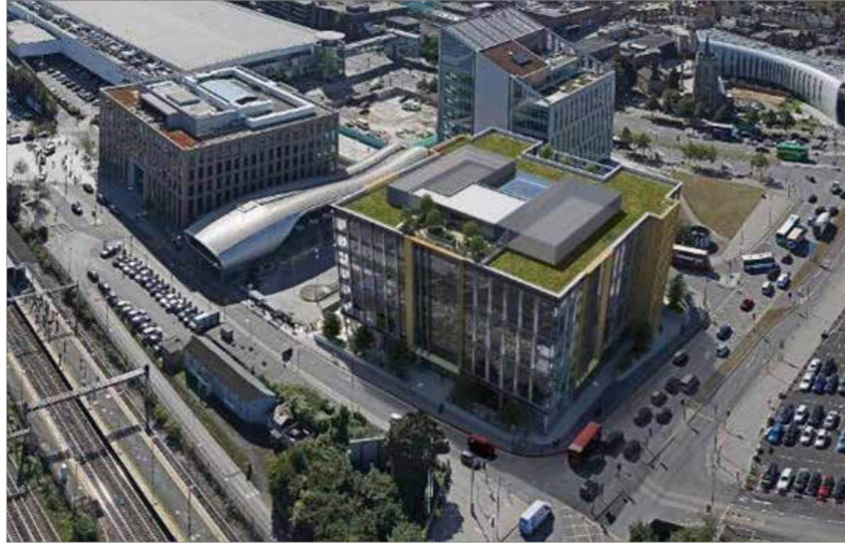
Figure 14: Station Quarter, Slough
