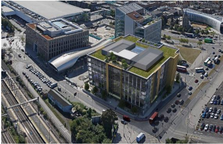
Figure 15: Station Quarter, Slough
